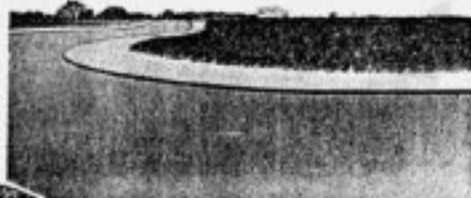
LOOKING WEST TOWARD SULLIVAN WAY
